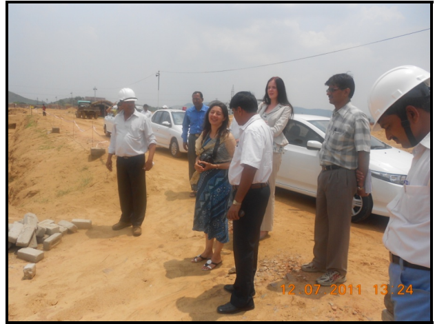
SAI India staff and INTOSAI WGEA representatives tour iCED construction site
