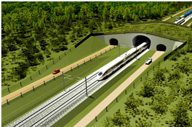
The ecoduct (wildlife crossing) of the Rail Baltica in the future.
